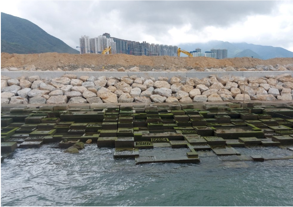
Photo 4 – Natural Rock Material/Planting for Artificial Seawall
