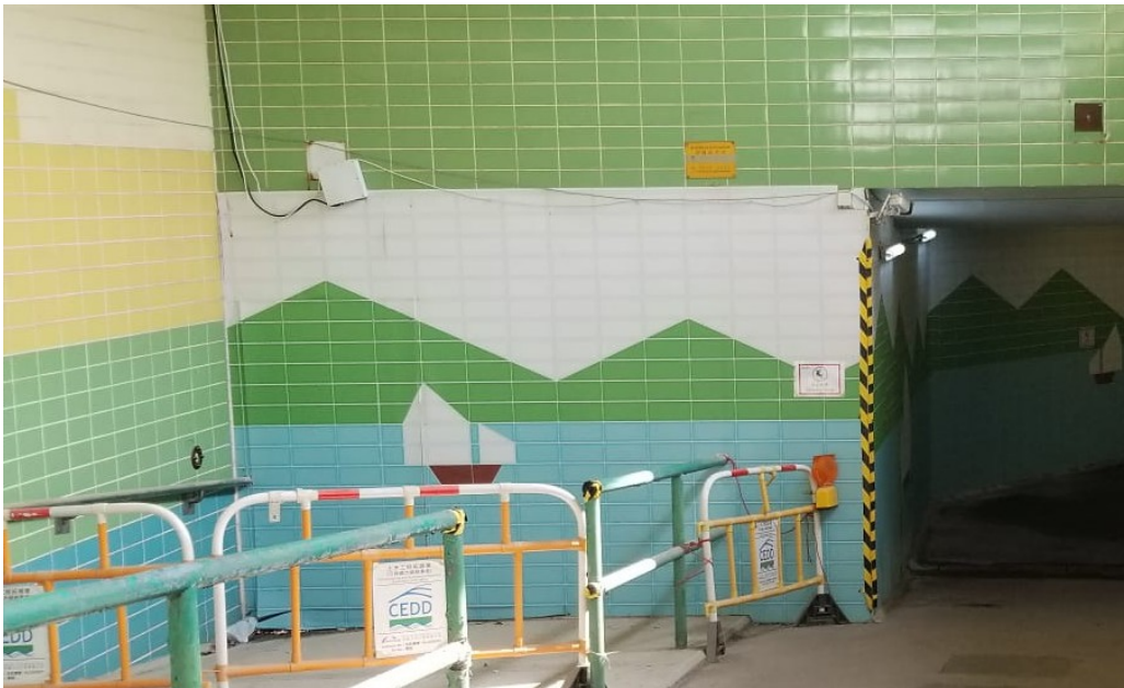
Photo 3 – Erection of site hoardings in unobtrusive colours
