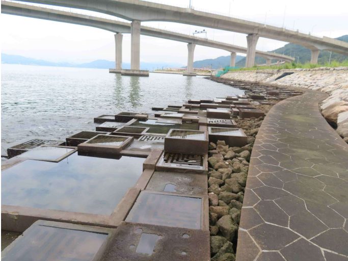
General View of Rocky Eco-shoreline
