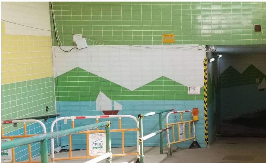
Photo 3 – Erection of site hoardings in unobtrusive colours
