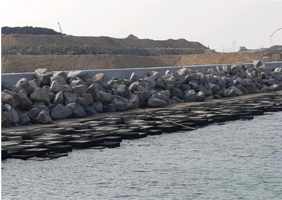
Photo 3 - Natural Rock Material/ Planting for Artificial Seawall
