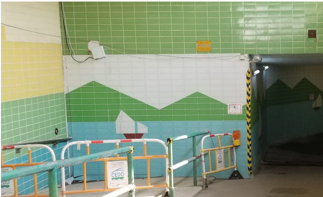
Photo 3 – Erection of site hoardings in unobtrusive colours
