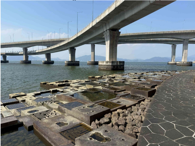
General View of Rocky Eco-shoreline
