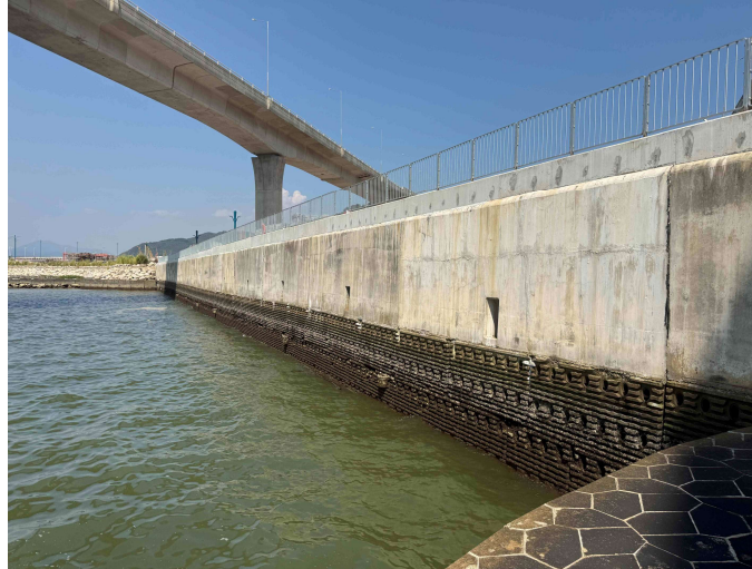
General View of Vertical Eco-shoreline
