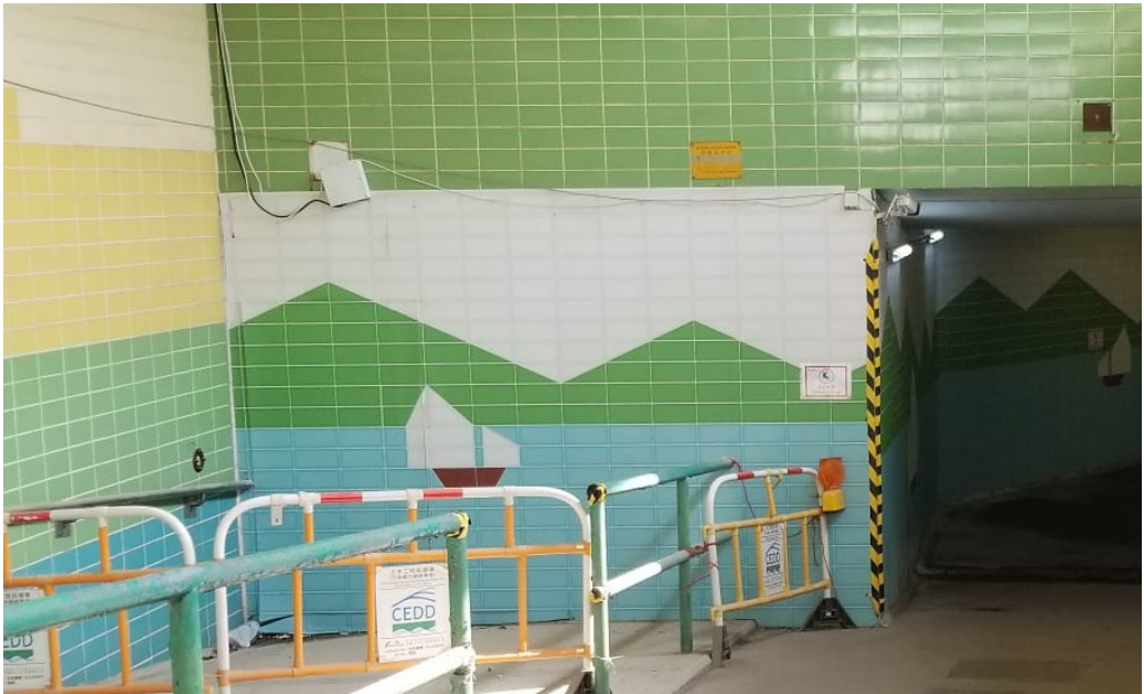
Photo 3 – Erection of site hoardings in unobtrusive colours
