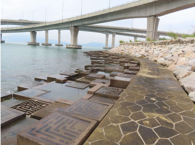
General View of Rocky Eco-shoreline
