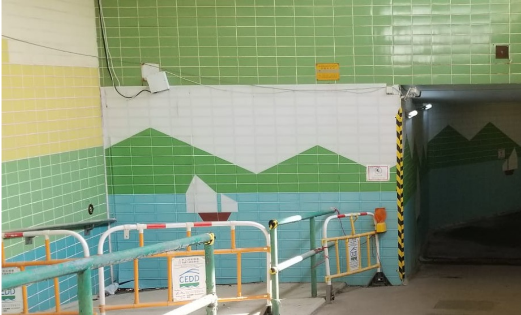
Photo 3 – Erection of site hoardings in unobtrusive colours
