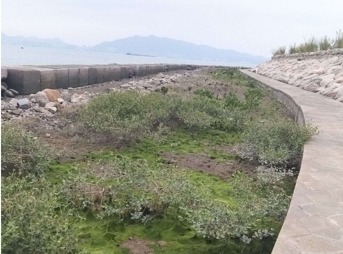
General View of Mangrove Eco-shoreline at Upper Terrace
