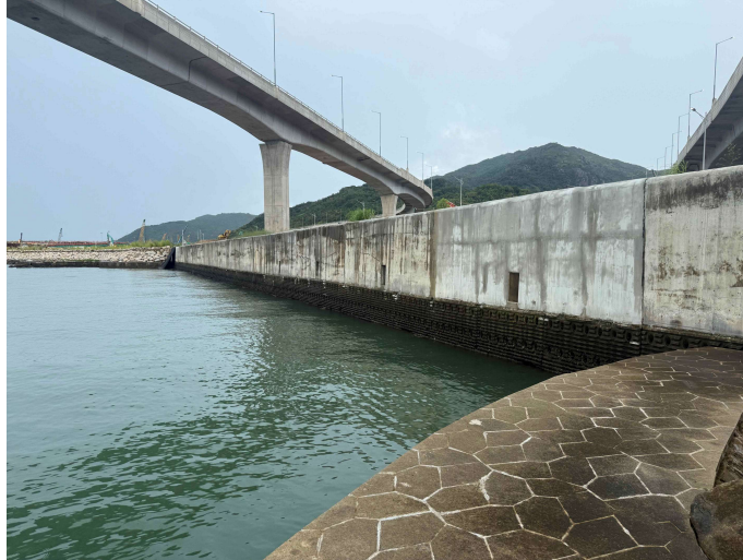
General View of Vertical Eco-shoreline
