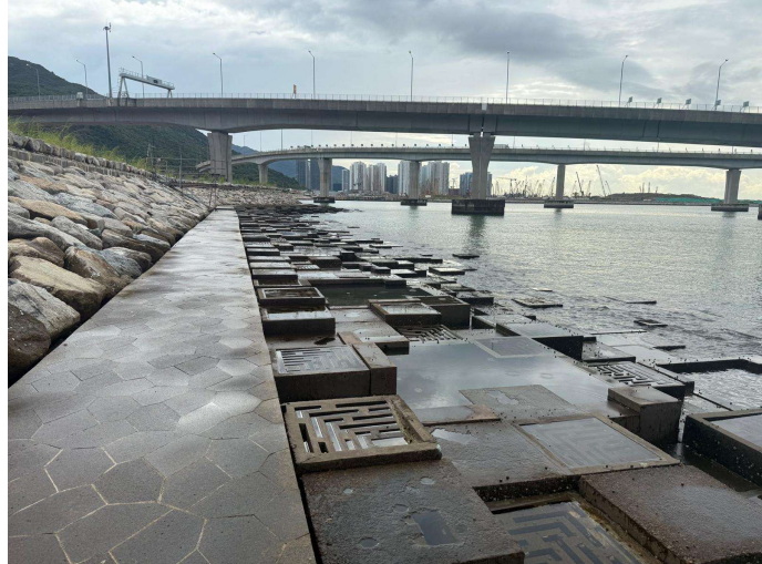
General View of Rocky Eco-shoreline
