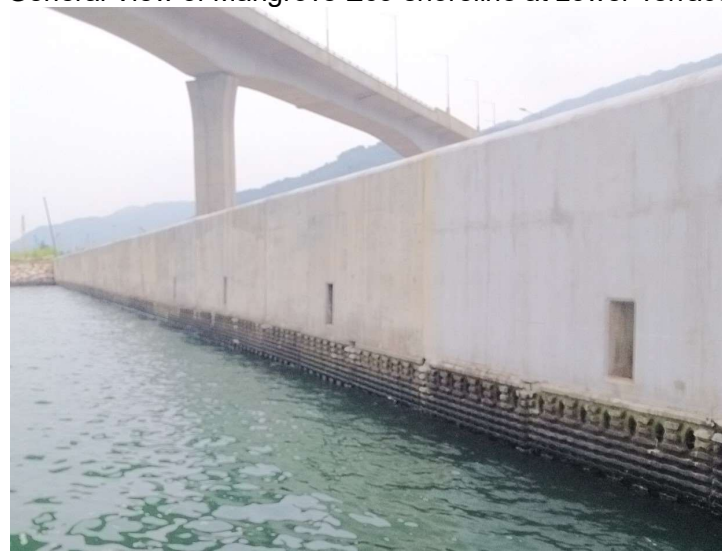
General View of Vertical Eco-shoreline
