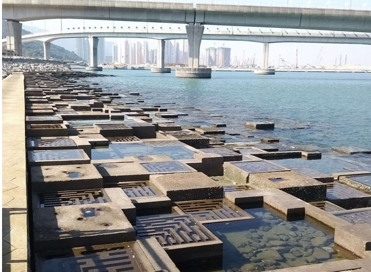
General View of Rocky Eco-shoreline
