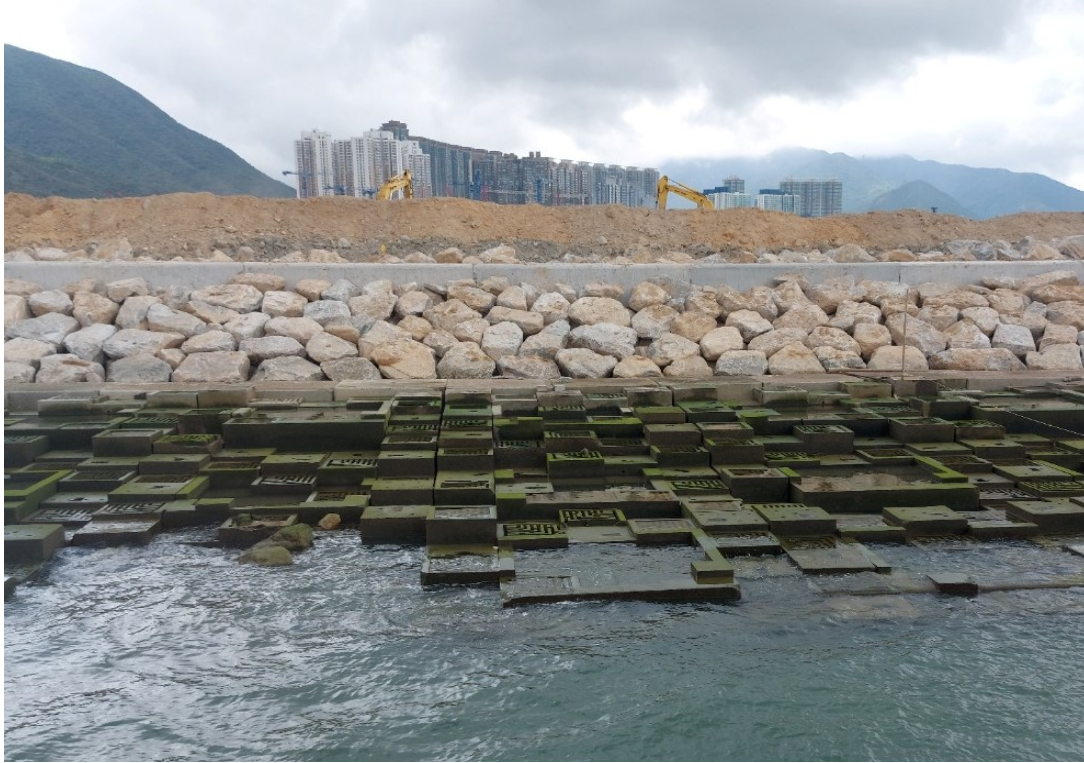
Photo 4 – Natural Rock Material/Planting for Artificial Seawall
