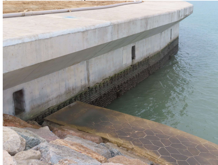
General View of Vertical Eco-shoreline
