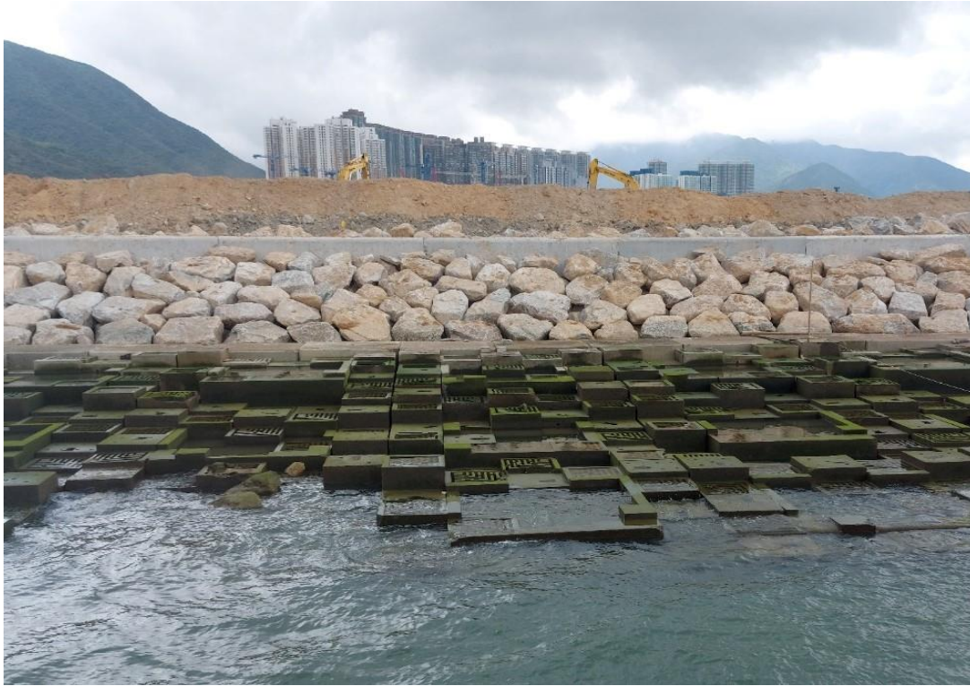
Photo 4 – Natural Rock Material/Planting for Artificial Seawall
