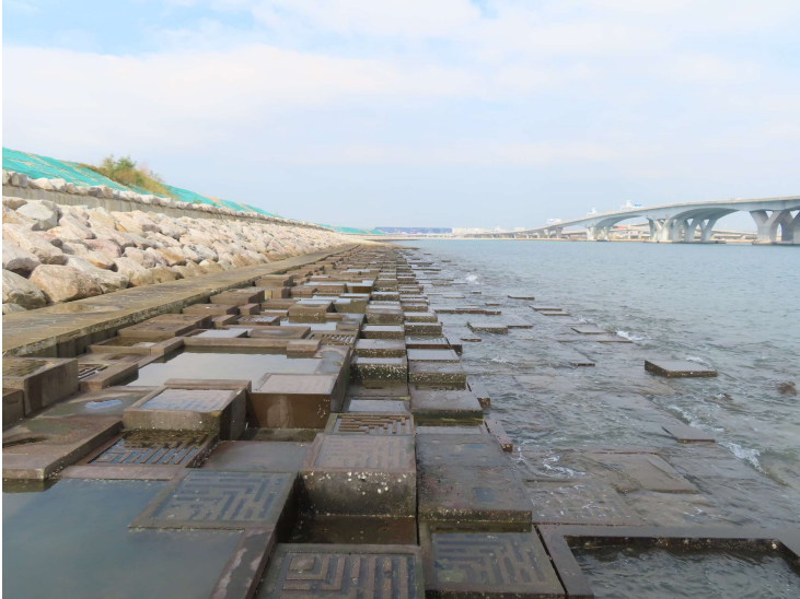
General View of Rocky Eco-shoreline
