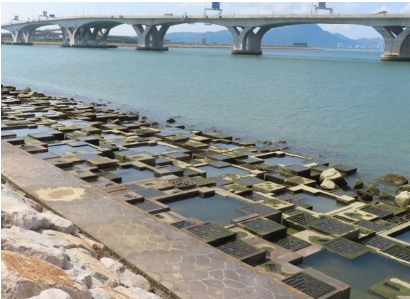
General View of Rocky Eco-shoreline
