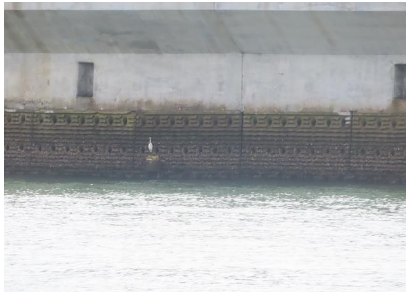
General View of Vertical Eco-shoreline
