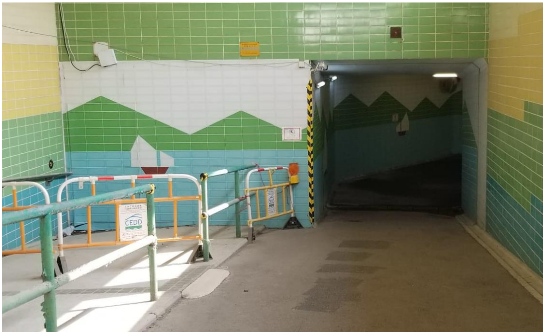
Photo 3 - Erection of site hoardings in unobtrusive colours
