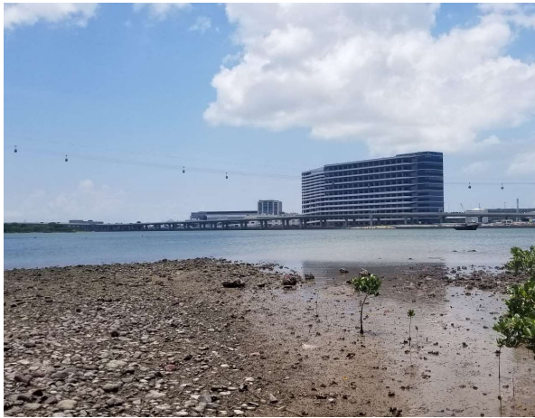
(a) Survey Location at TCB1
