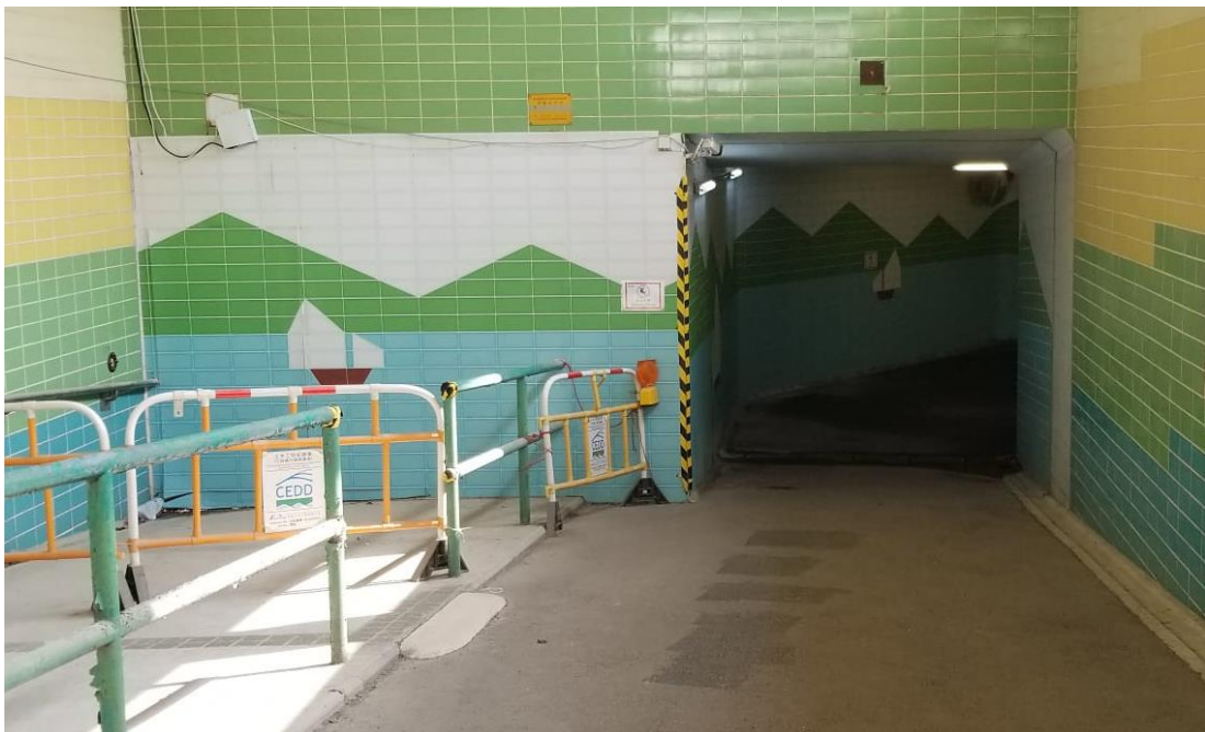
Photo 3 - Erection of site hoardings in unobtrusive colours
