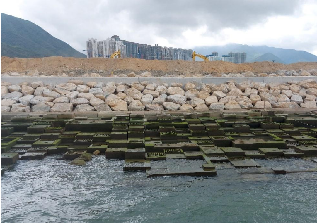
Photo 4 – Natural Rock Material/Planting for Artificial Seawall
