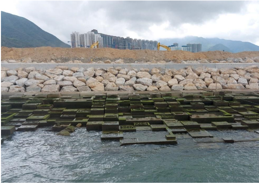
Photo 4 – Natural Rock Material/Planting for Artificial Seawall
