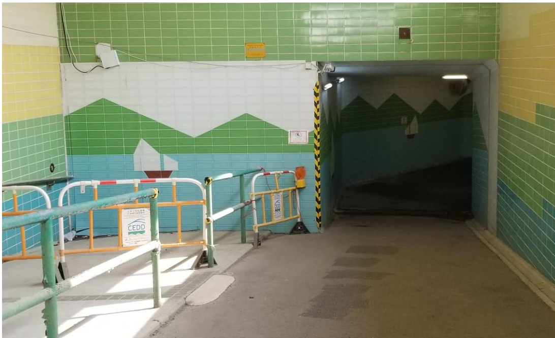
Photo 3 - Erection of site hoardings in unobtrusive colours
