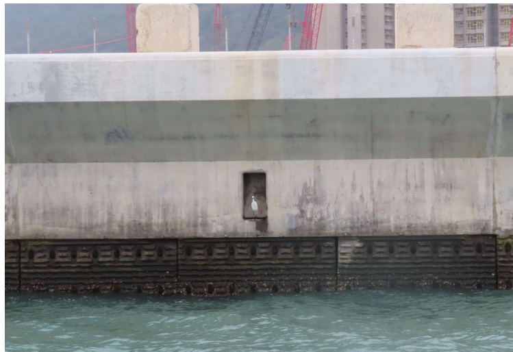
General View of Vertical Eco-shoreline
