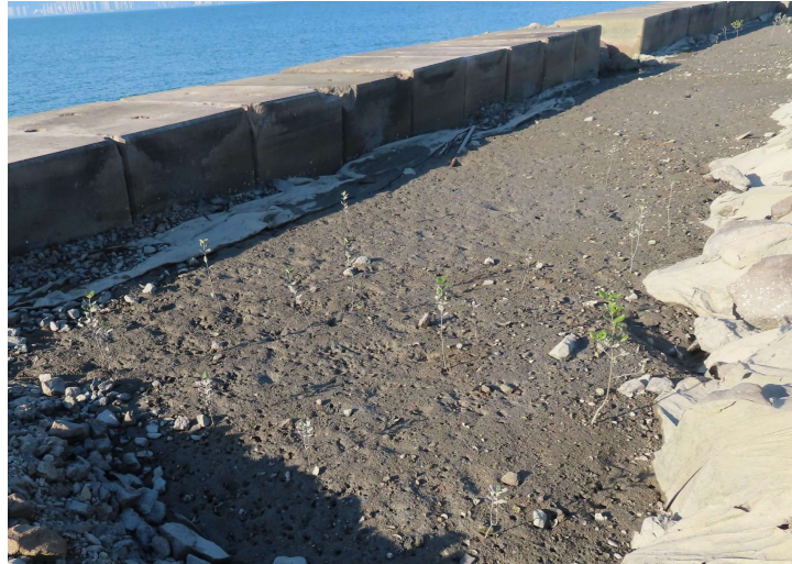
General View of Mangrove Eco-shoreline Lower Terrace
