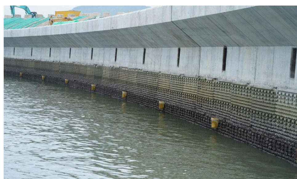
General View of Vertical Eco-shoreline
