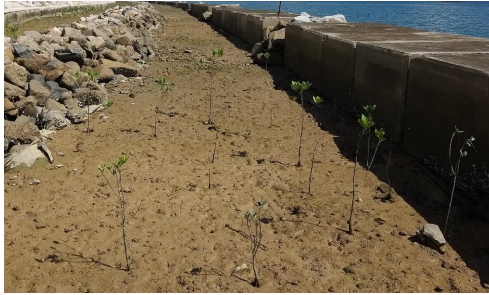
General View of Mangrove Eco-shoreline Lower Terrace
