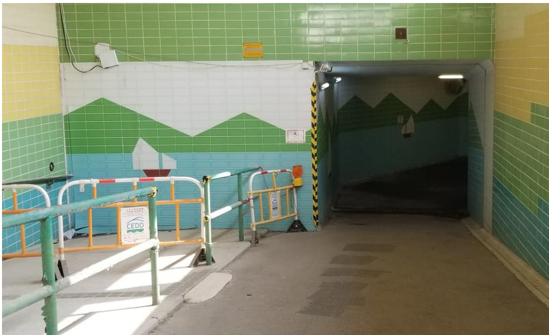
Photo 3 – Erection of site hoardings in unobtrusive colours
