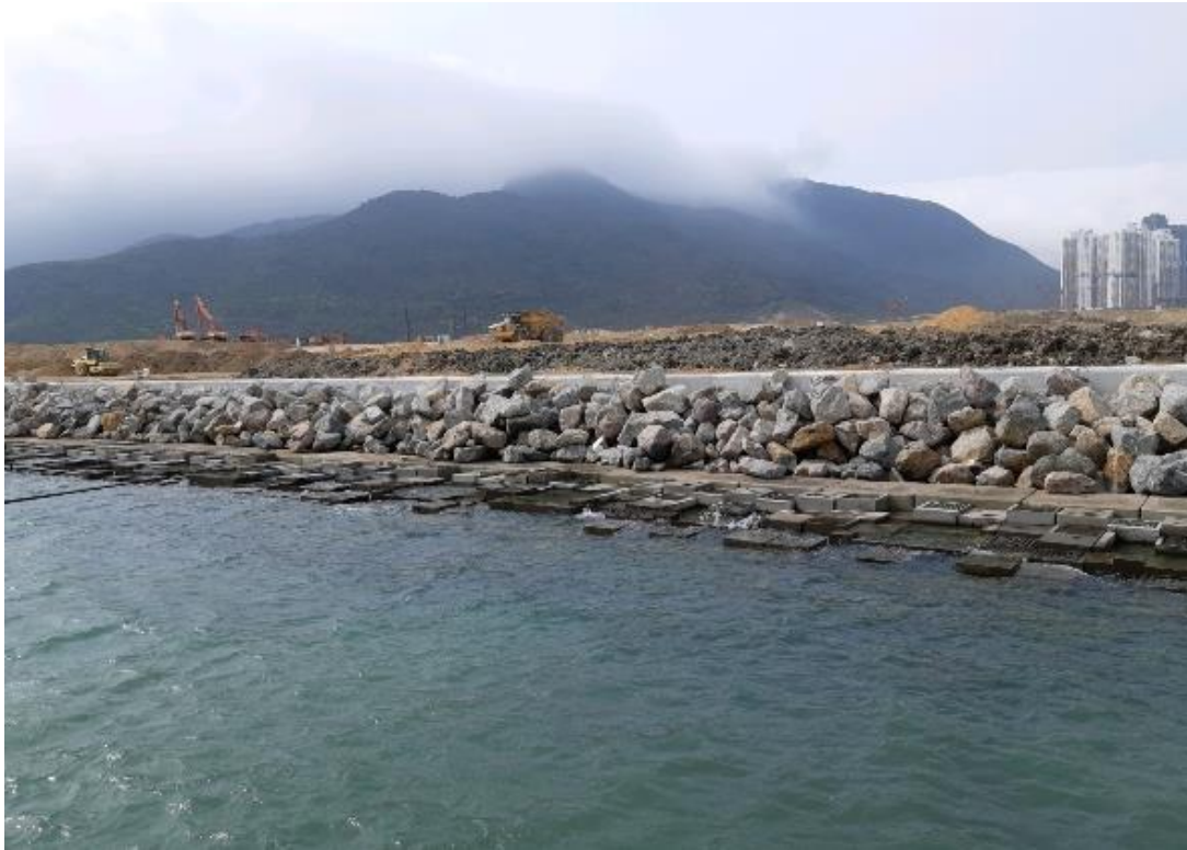
Photo 4 - Natural Rock Material/Planting for Artificial Seawall
