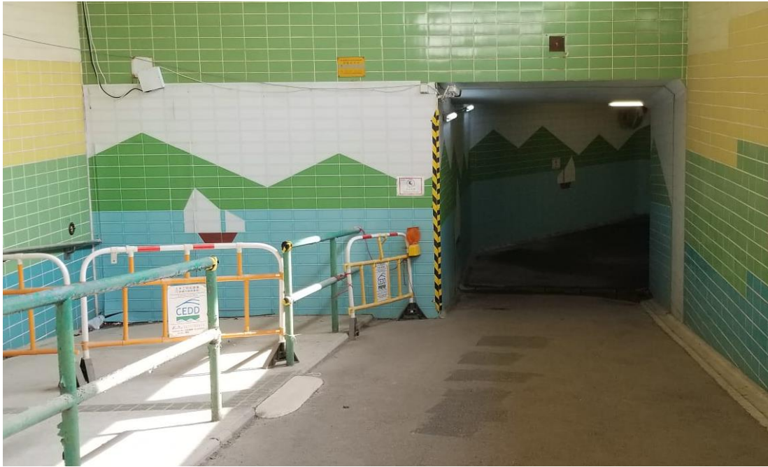
Photo 3 - Erection of site hoardings in unobtrusive colours
