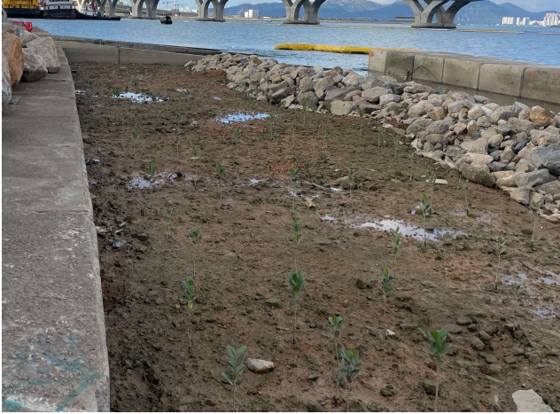
General View of Mangrove Eco-shoreline
