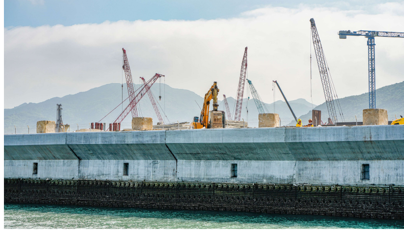
General View of Vertical Eco-shoreline
