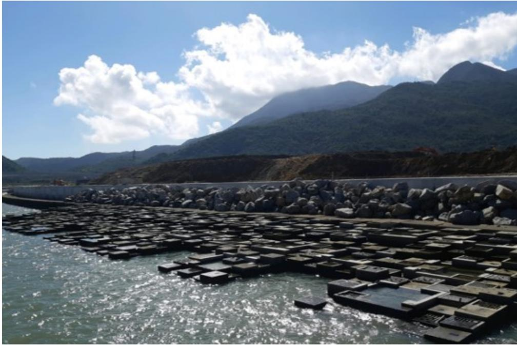
Photo 3 - Natural Rock Material/ Planting for Artificial Seawall
