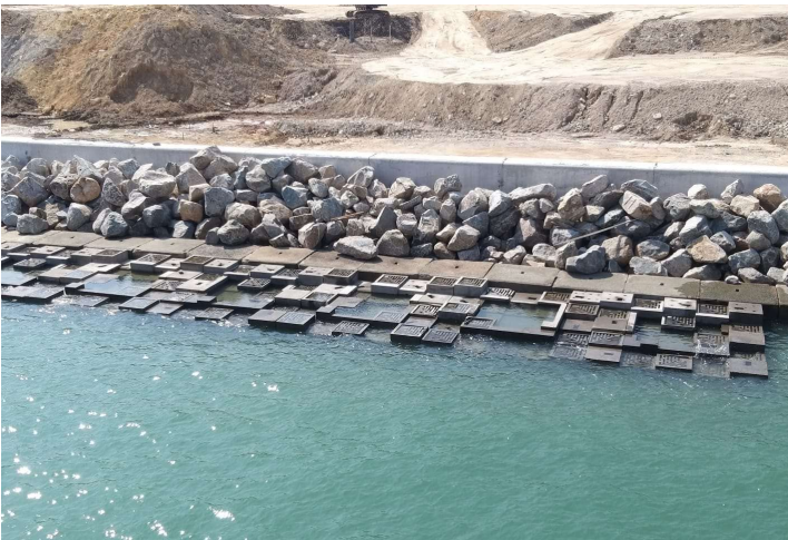
General View of Rocky Eco-shoreline
