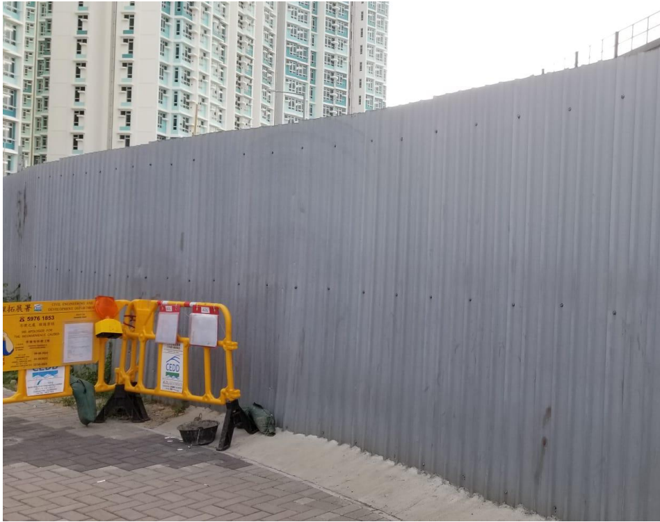
Photo 3 - Erection of site hoardings in unobtrusive colours
